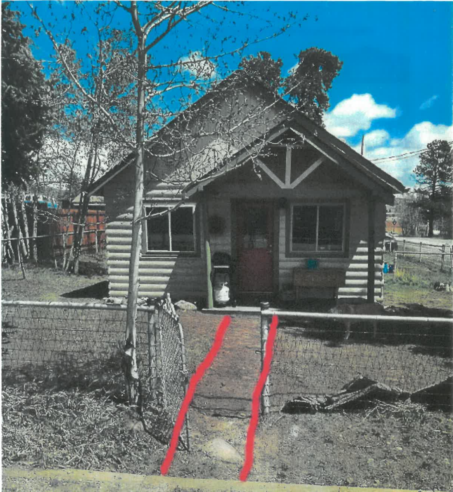
Flagstone Walk-way Installation Area (view from Bogue Street)
