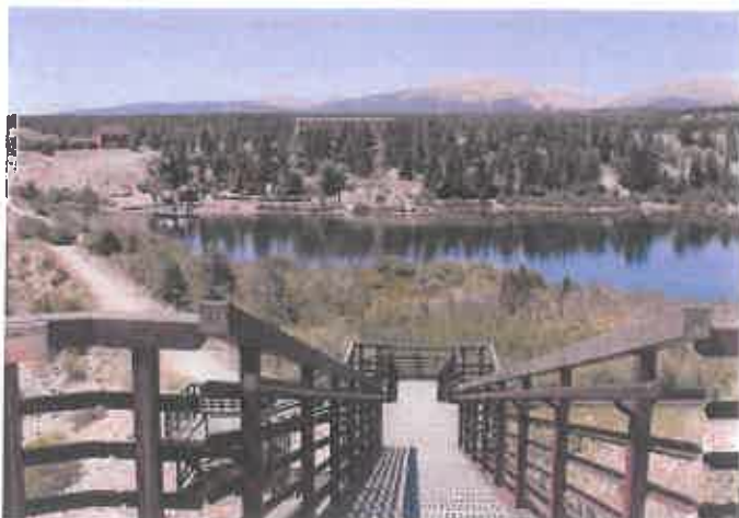
Existing steel stair connection to downtown
