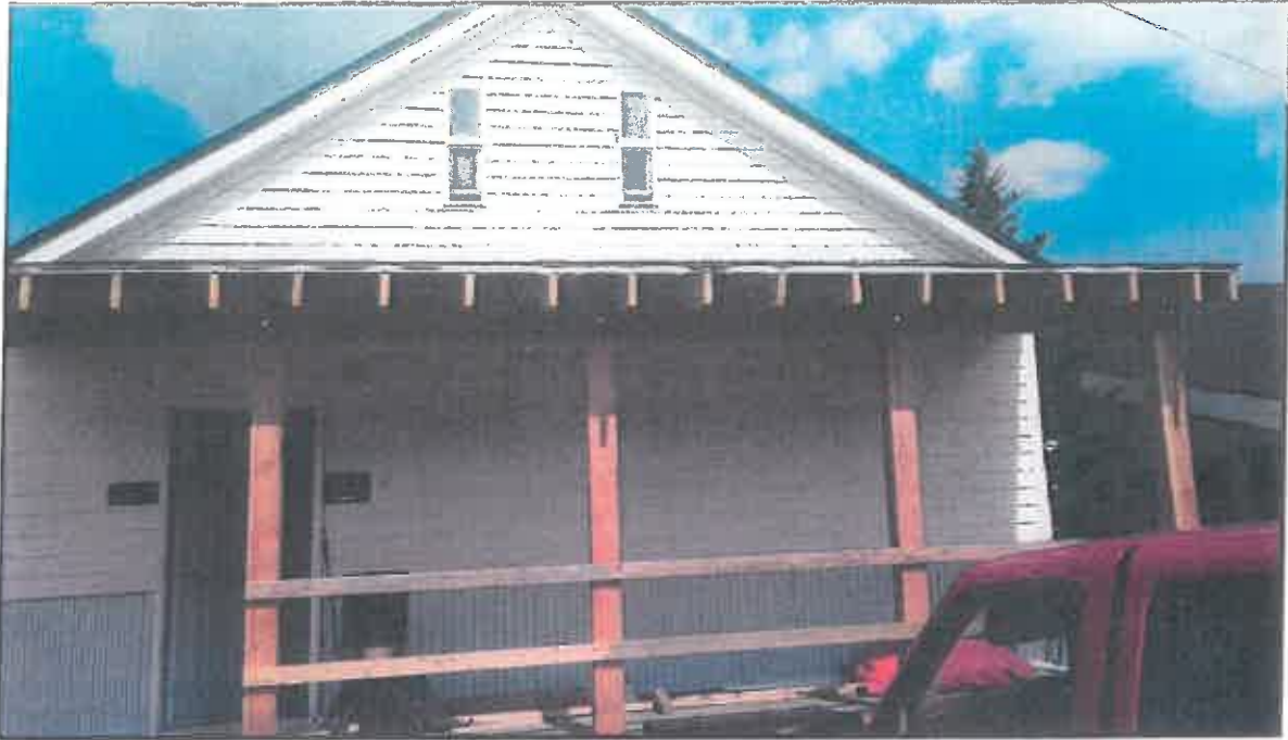
6 th Street Elevation Looking West
