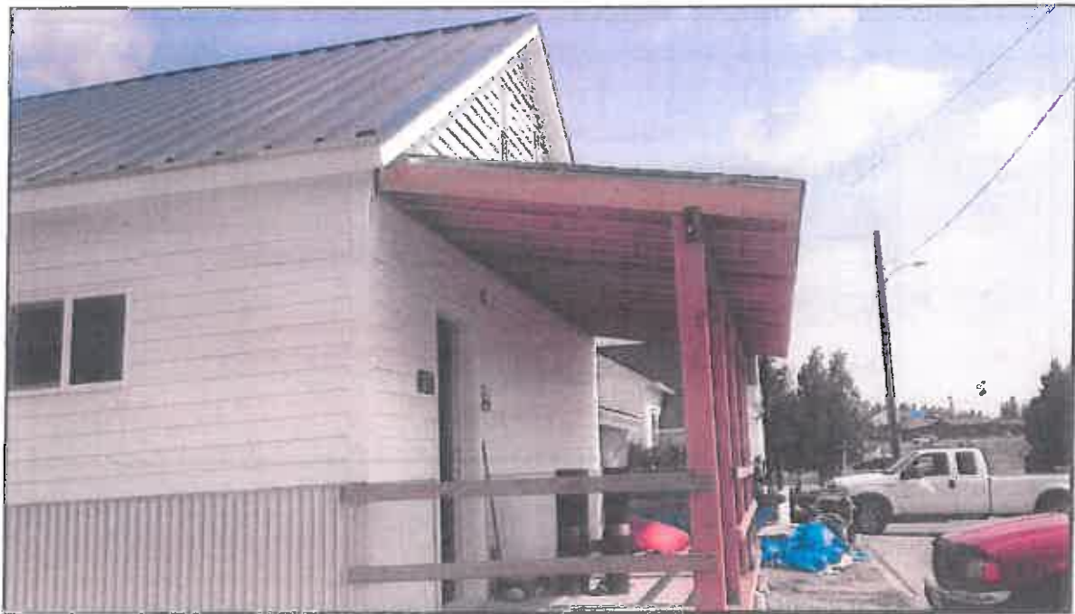
South Elevation Looking North
